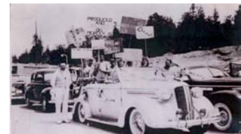
Cars waiting to cross the floating bridge for the first time!
